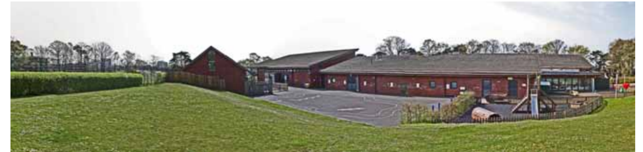
View to south towards two classroom block, the existing school and playground.
